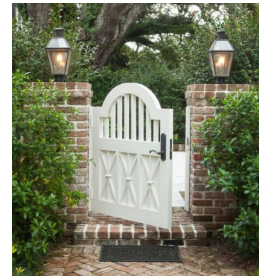
Gate with brick columns and lanterns
